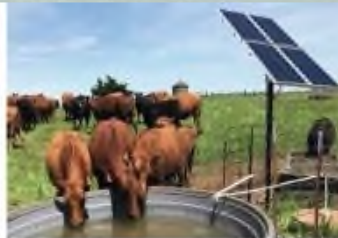
PV-powered dairy system
