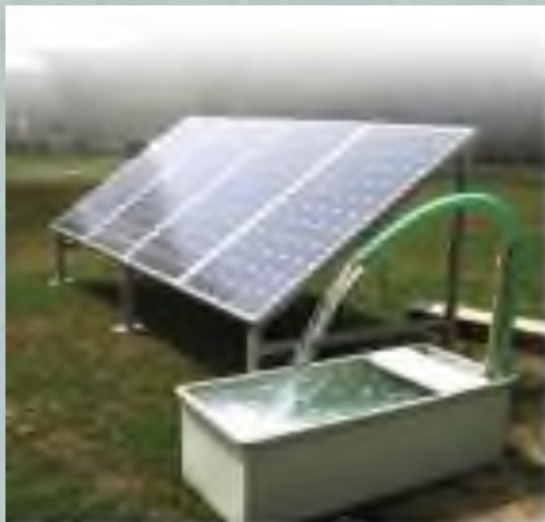
PV-powered pumping system
