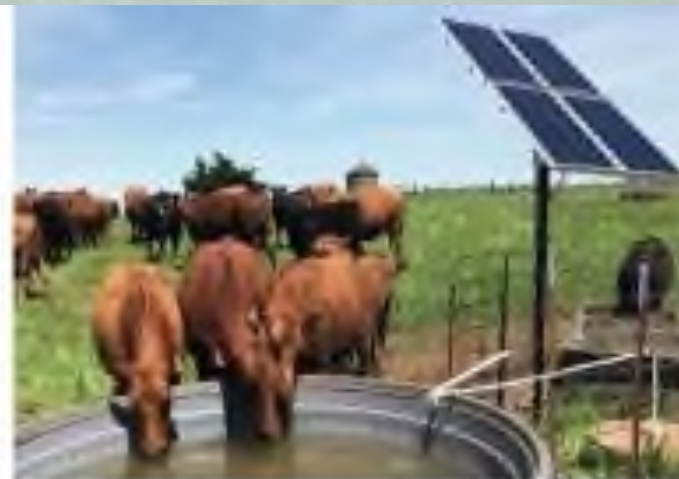
PV-powered dairy system
