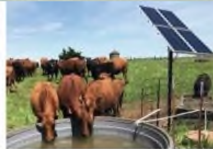
PV-powered dairy system
